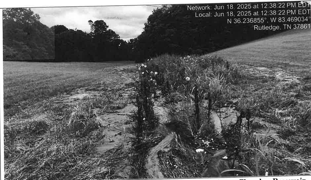
Photo 2: Sediment deposits in wet weather conveyance that drains to Cherokee Reservoir.
